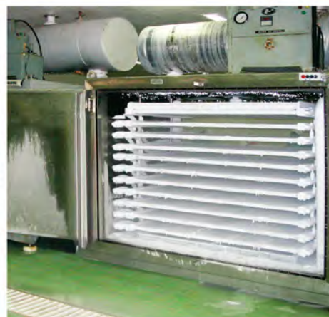
Ice bank coil NIB-C Thermal storage capacity range 122 to 305 kw.hr
