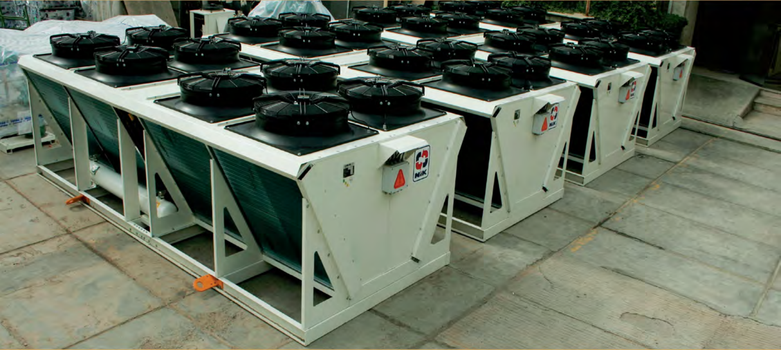
Air cooled v-type condenser NGV Capacity range 64.8 to 838.3 kW Fan diameter 630, 710 or 800 mm NO. of fans 2 up to 14 fans
