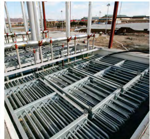
Freon prefabricated ice bank NIB-F Thermal storage capacity range 90 to 450 kw.hr
